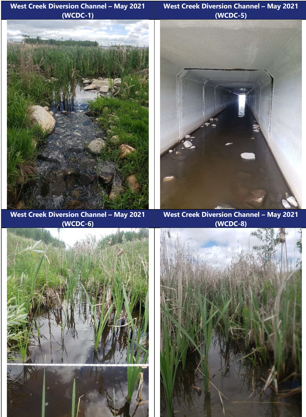
Photo B-4: West Creek Diversion Channel (upstream of haul road), May 2021
