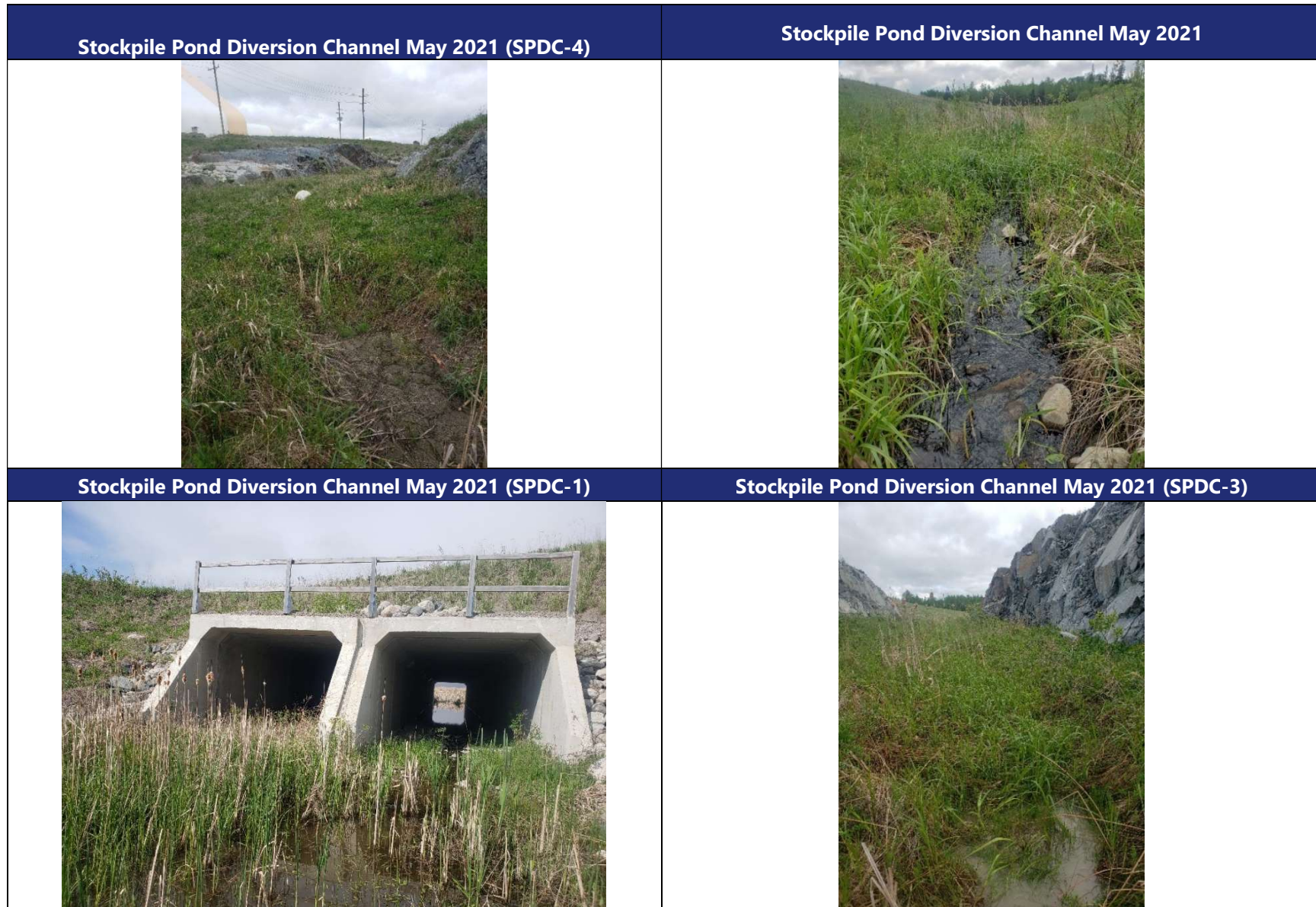
Photo B-1: Stockpile Pond Diversion Channel Habitat, May 2021
