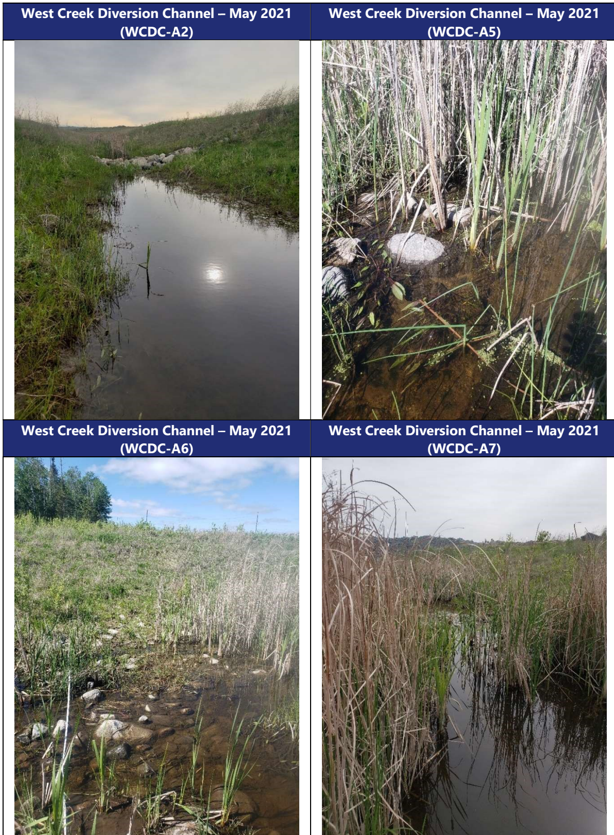
Photo B-5: West Creek Diversion Channel (downstream of haul road), May 2021
