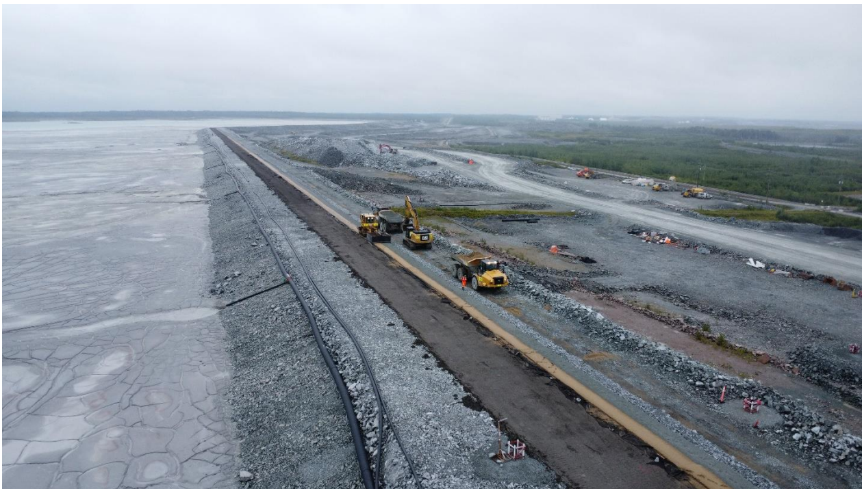
Figure 10. TMA Dam construction during filter placement, 2024
