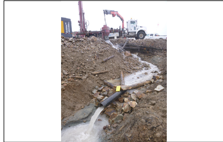
PHOTO 2 – PW13-1 discharge measurement
