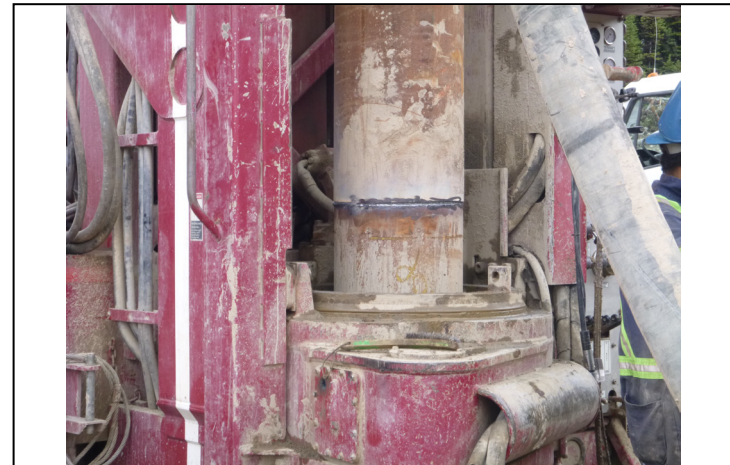
PHOTO 4 – 16 inch casing weld, PW13-3
