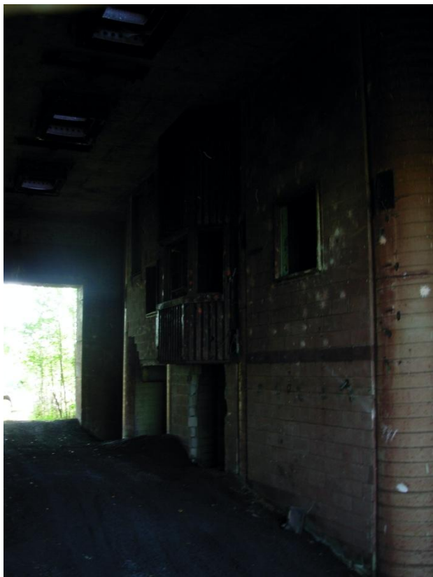
Inside Rail Load-out Silo
