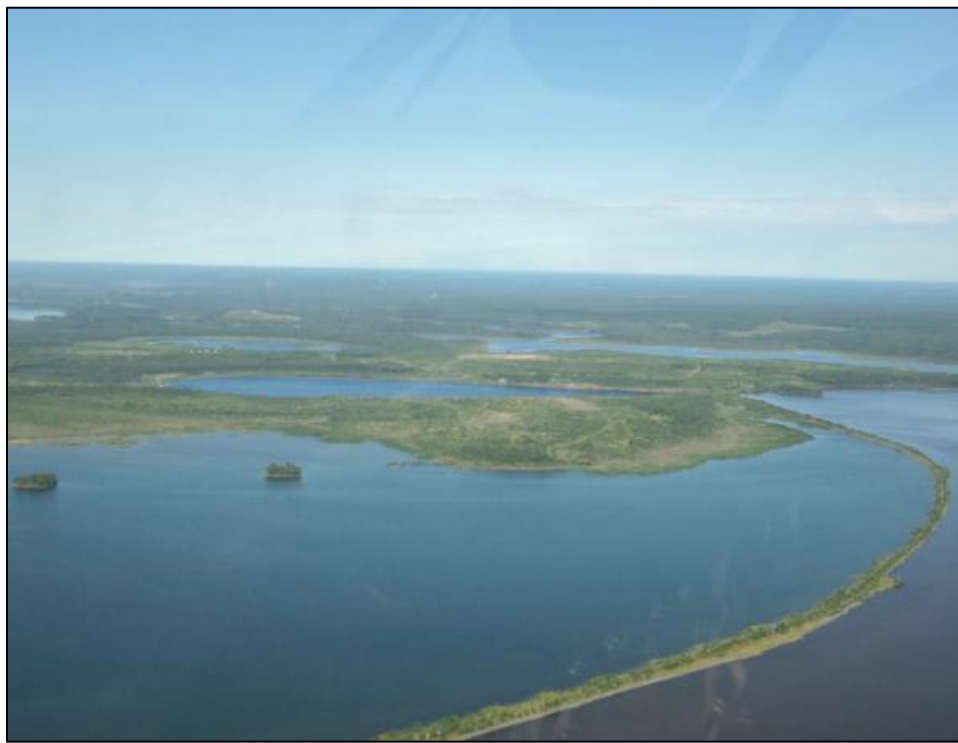
Photograph 13: Existing Perimeter Dyke
