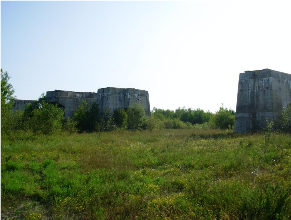
Kiln Foundation Looking Northeast
