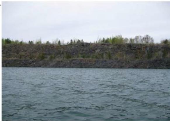
8 Portion of North pit wall. Note that water level has almost reached the top bench level.
