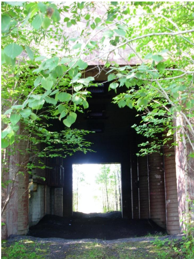
Rail Load-out Silo Looking South
