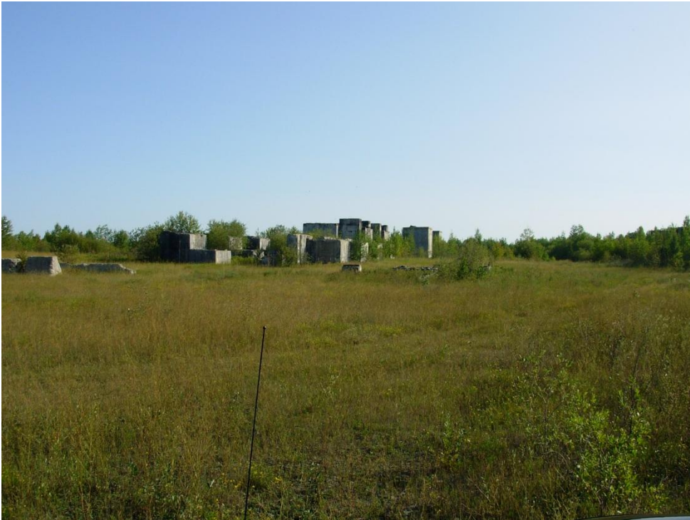
Concentrator Foundations Looking North
