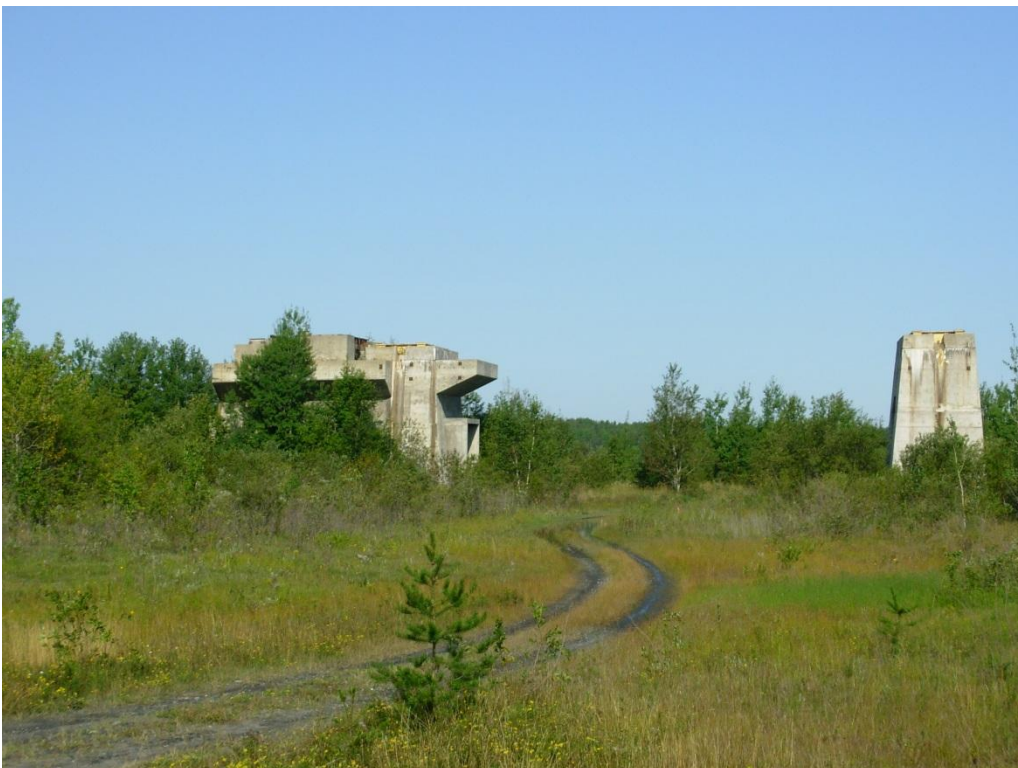
Kiln Foundation Looking West
