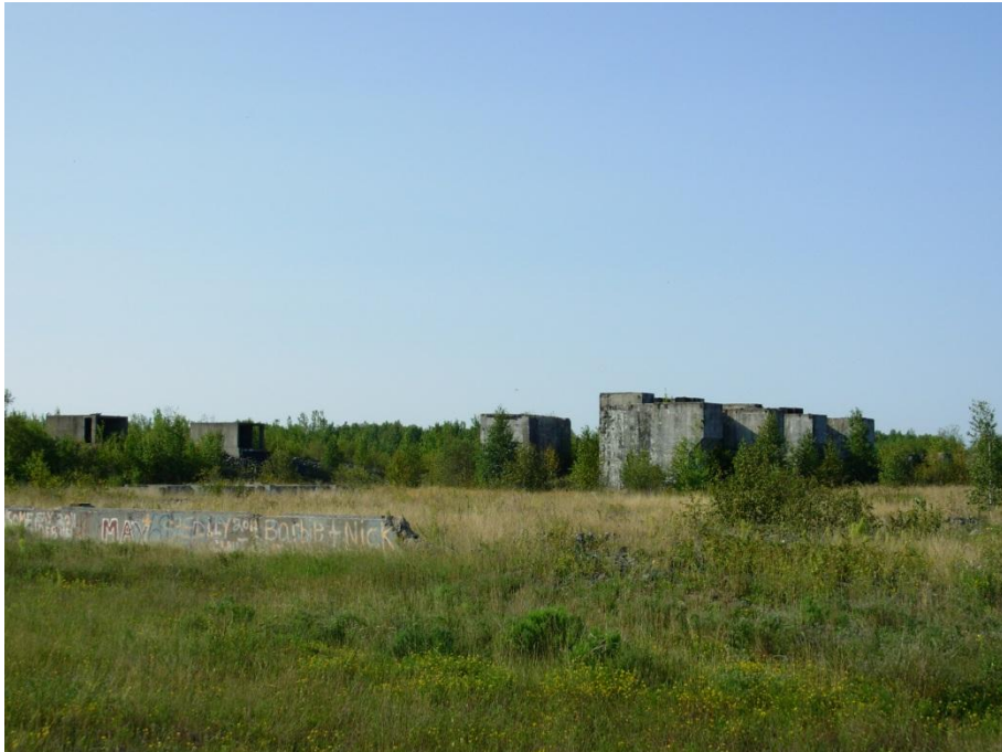
Plant Foundation Looking South
