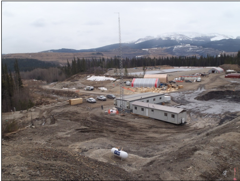
Plate 3.9-7. Eastern view of the Decline Site area facing south (April 2014).
