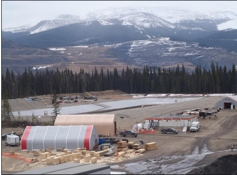
Plate 3.9-9. Lined sediment pond in the southeastern part of the Decline Site area (April 2014).
