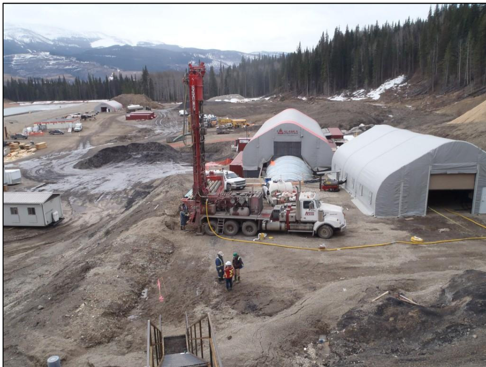
Plate 3.9-8. Western view of the Decline Site area facing south (April 2014).
