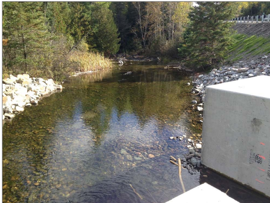
Plate 8: Borden River downstream of culverts on Highway 101 (October 2015)
