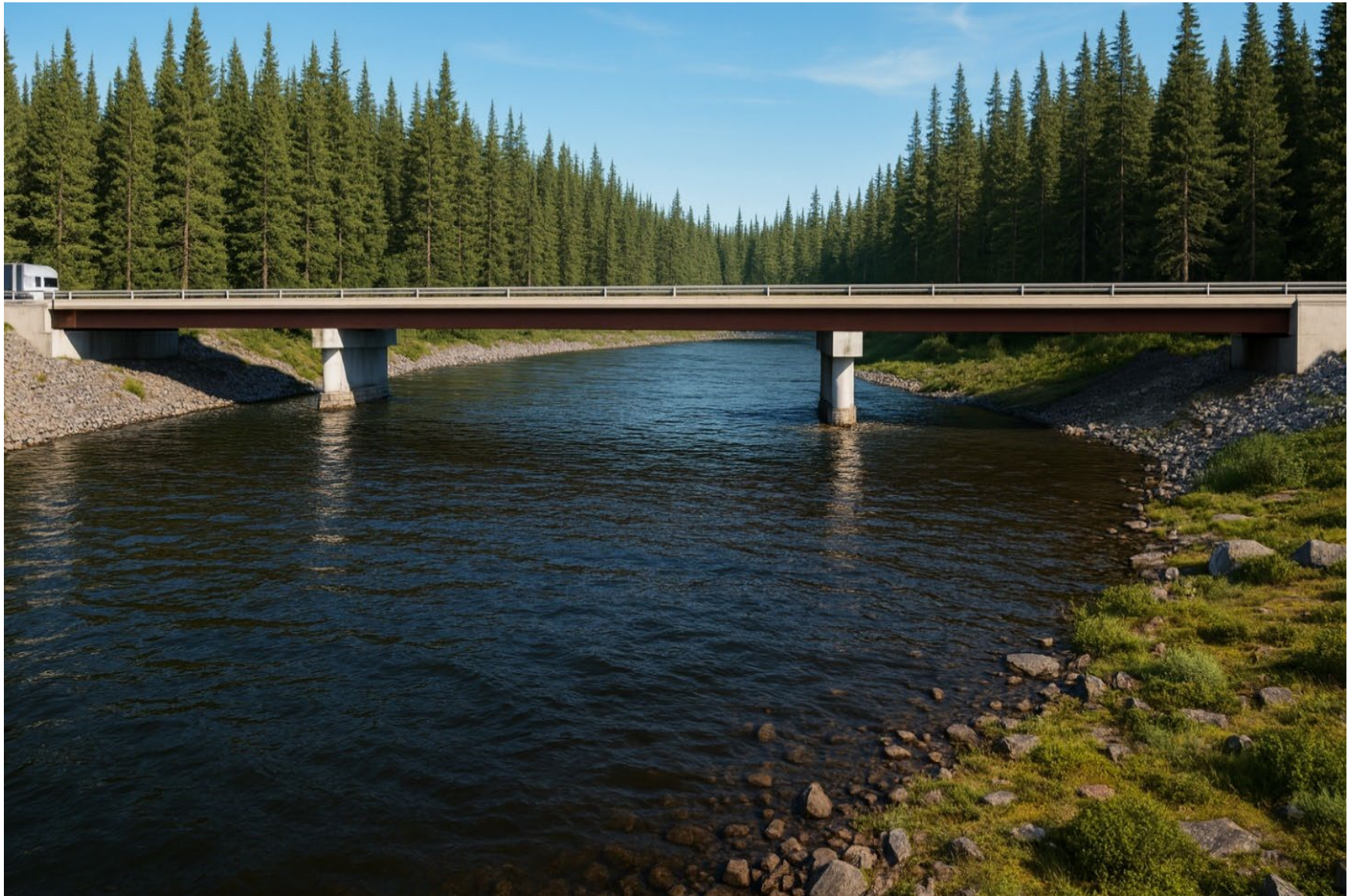
Figure 7-10: Crossing WA15 – Albany River
