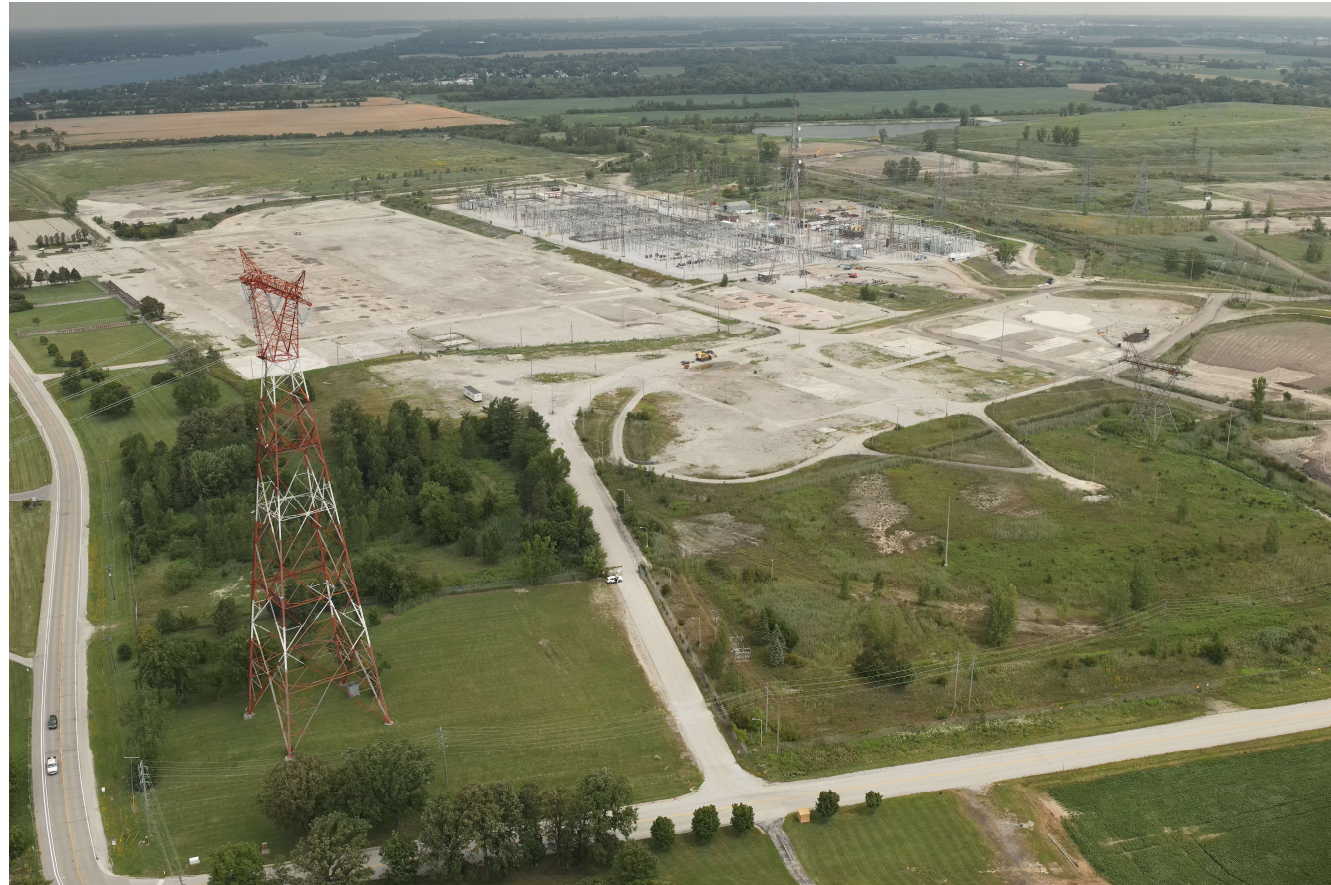
Pictured: Aerial view of the site.
