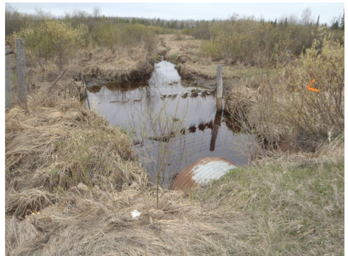
Photo 32: On Highway 600 road crossing, facing downstream, at MARR-4, on Marr Creek.
