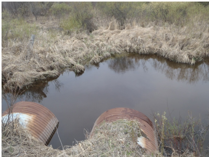
Photo 31: On Highway 600 road crossing, facing upstream, at MARR-4, on Marr Creek.
