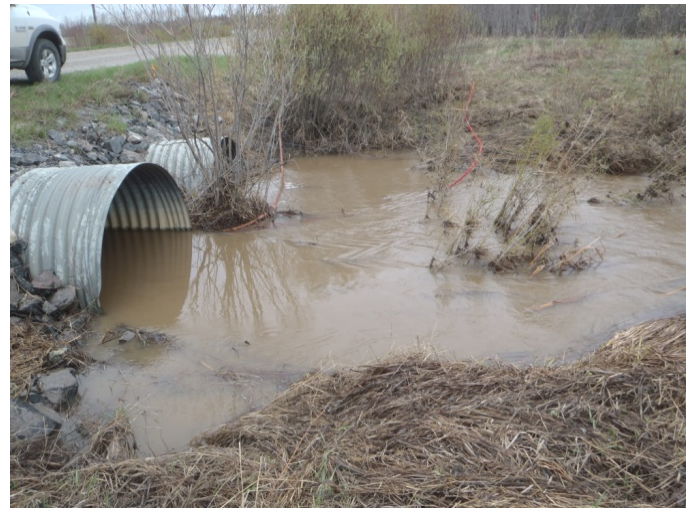
Photo 38: Culverts at Highway 600 road crossing, at CLA-4, on Clark Creek.
